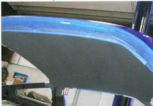
21 Headliner installation is complete. The small pieces of wind lace need to remain in place until the windshield and backlite are installed.
